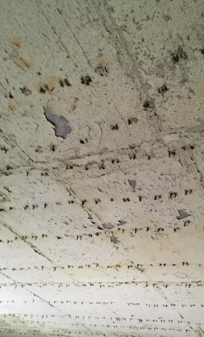
Plastic Chairs in Sulfur pit melted after operation
